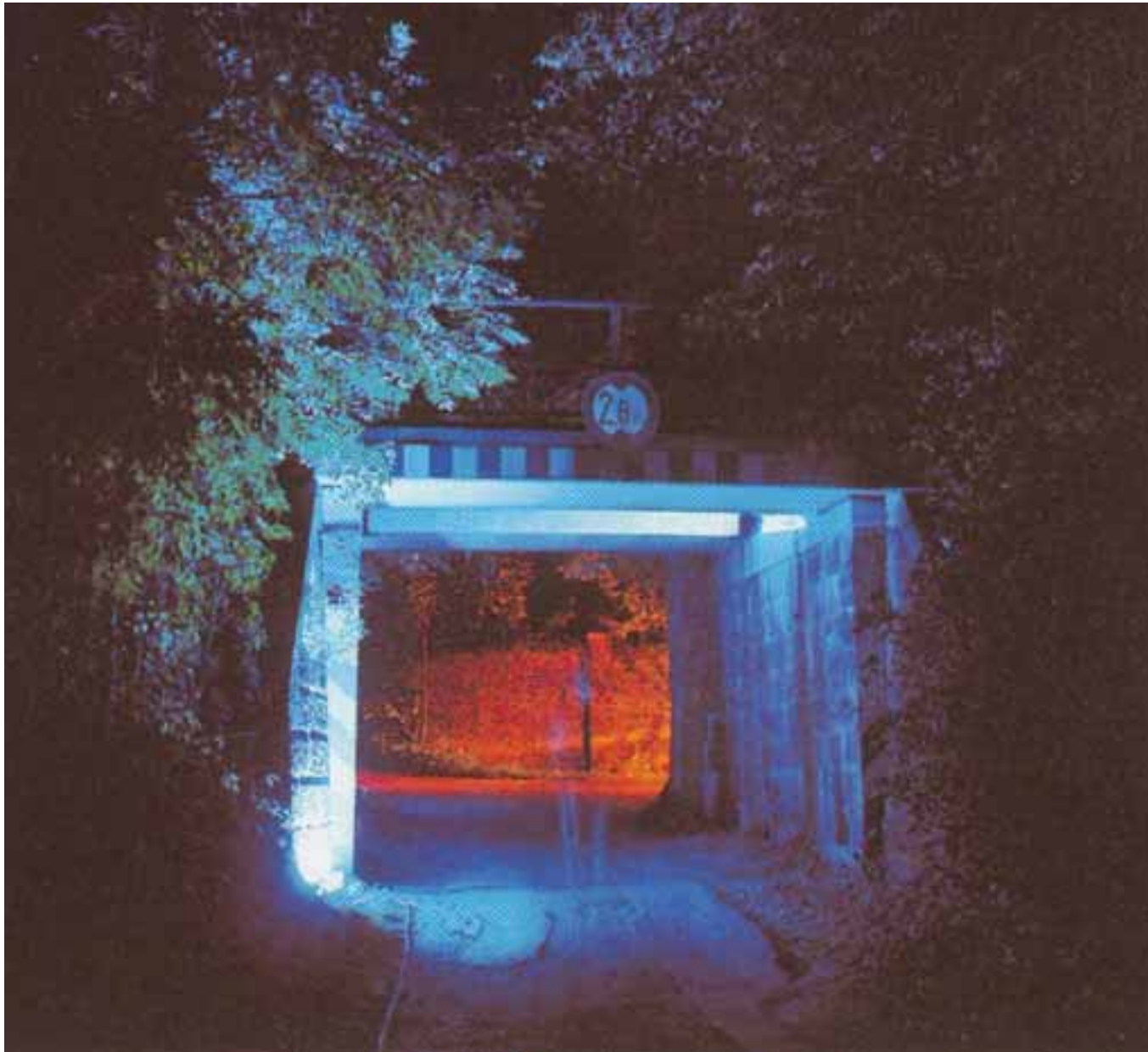
Lichtinstallation in Tunnel
